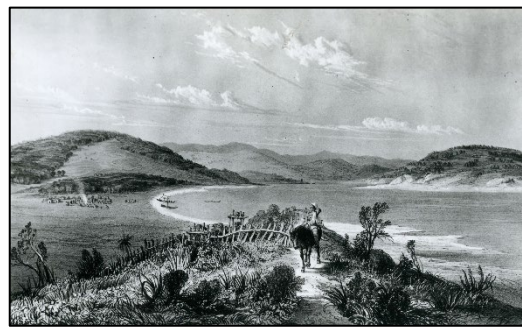
View of Taupō Kainga from the Taua Tapu Track. 238
