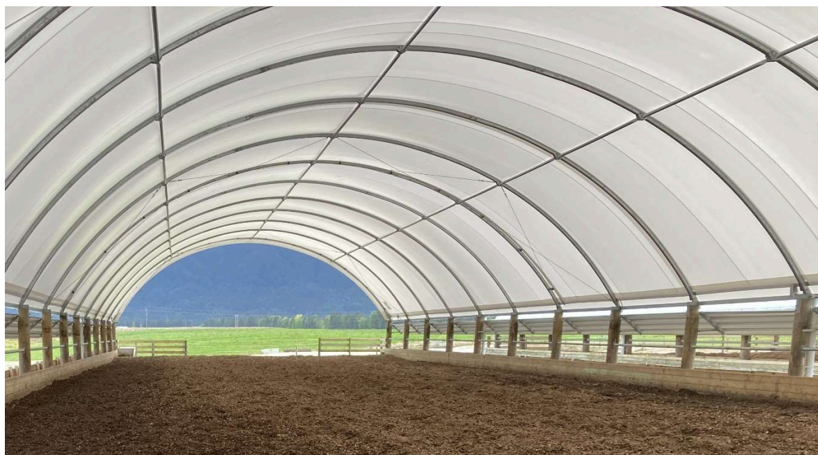
Figure 20. Photo of the Mootel roof at Turkey Creek farm
