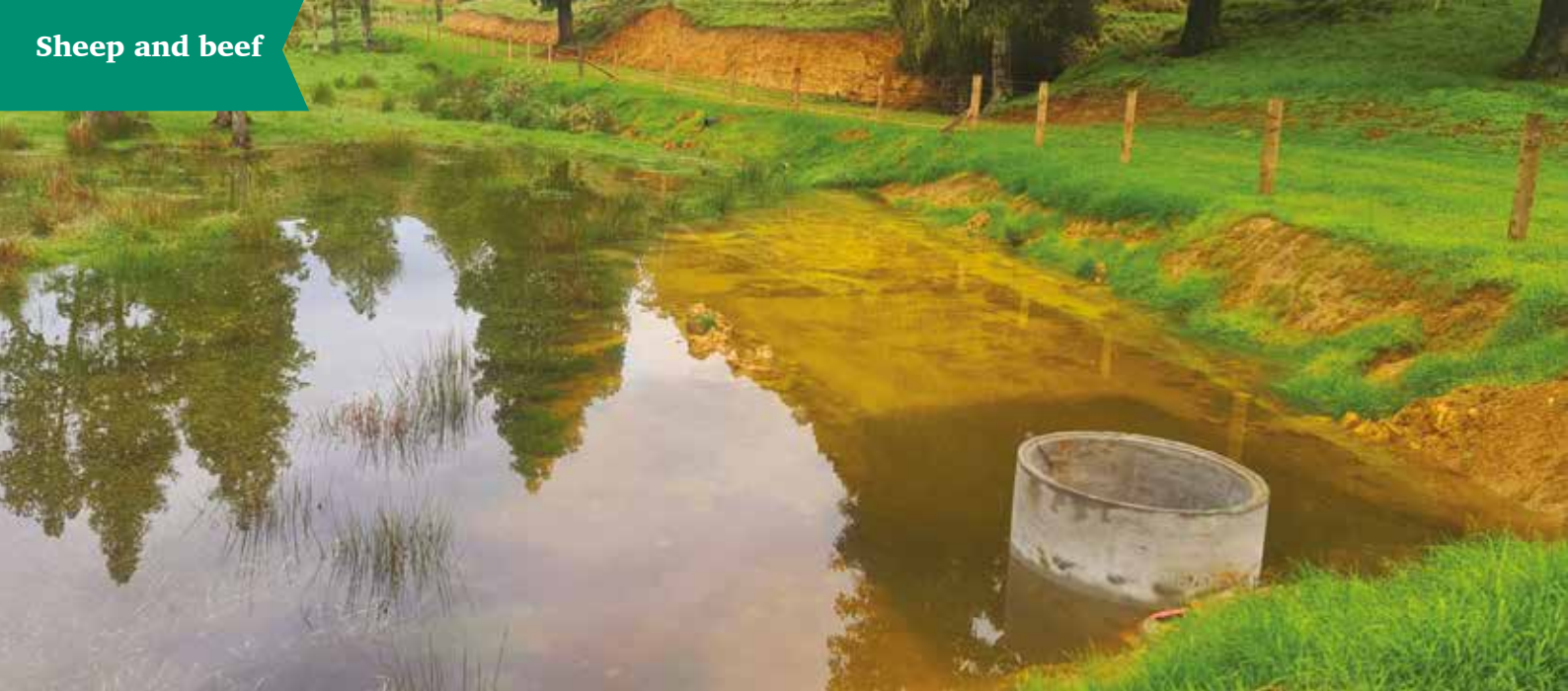
Sediment trap at Russell Proffit's farm
