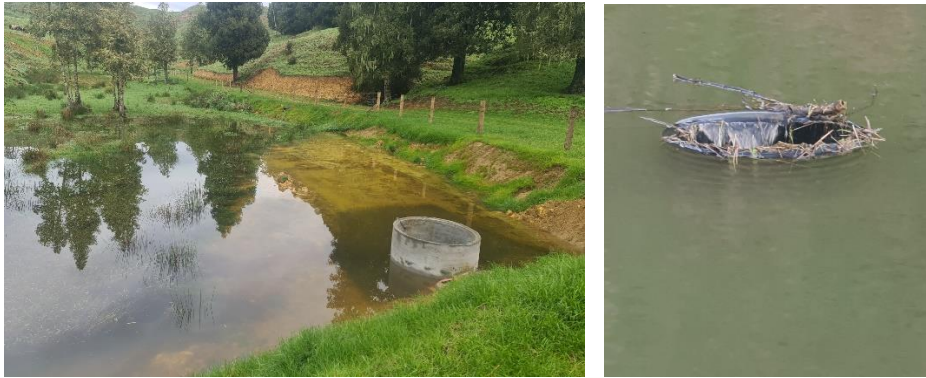
Figure 1. Sediment trap at one of the properties in the study (left) and example of an upstanding riser trialled in the study (right).
